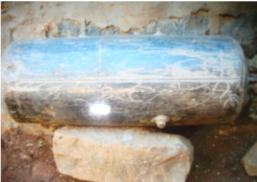
Plate 1: Steam storage system before lagging
